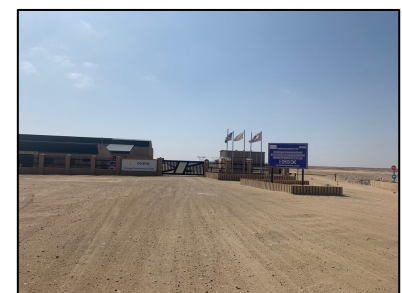
Figure 4. Arongo desalination plant
