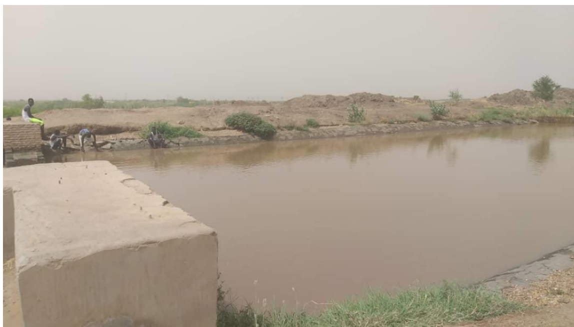
Figure 9: Main Irrigation Channel for Food Security Project at Al Damar
