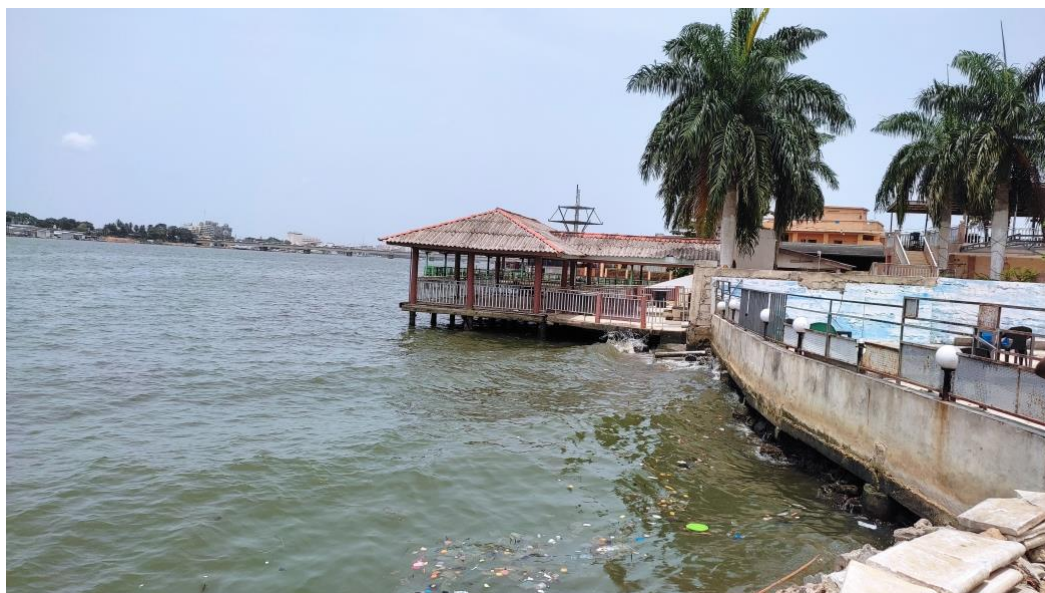
Fig. 11 - BARGE LAGUNAIRE OCCUPEE A BLOCKHAUSS
