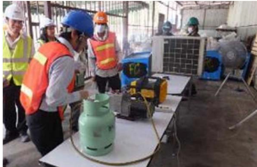
Demonstration for Recovery from Air- Conditioner
