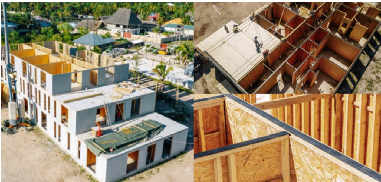
Construction using mass timber in Fumba Town: Photo by CPS
