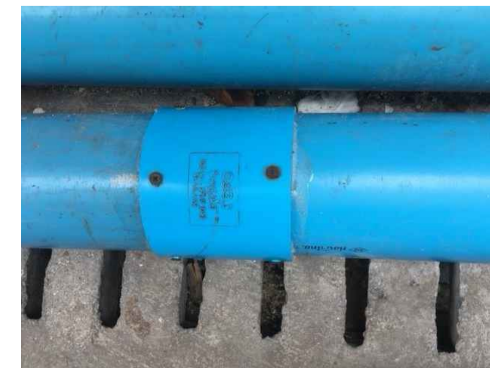
TYPICAL LOW PRESSURE PIPE JOINTING
