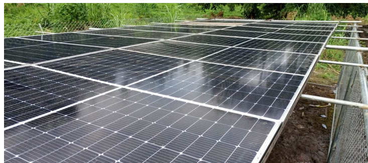
Figure 19: PV panels installed on Support structure.
