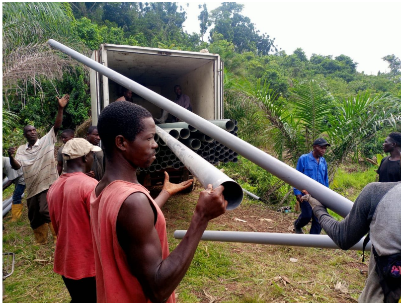
Figure 14: Offloading of pipes at site.
