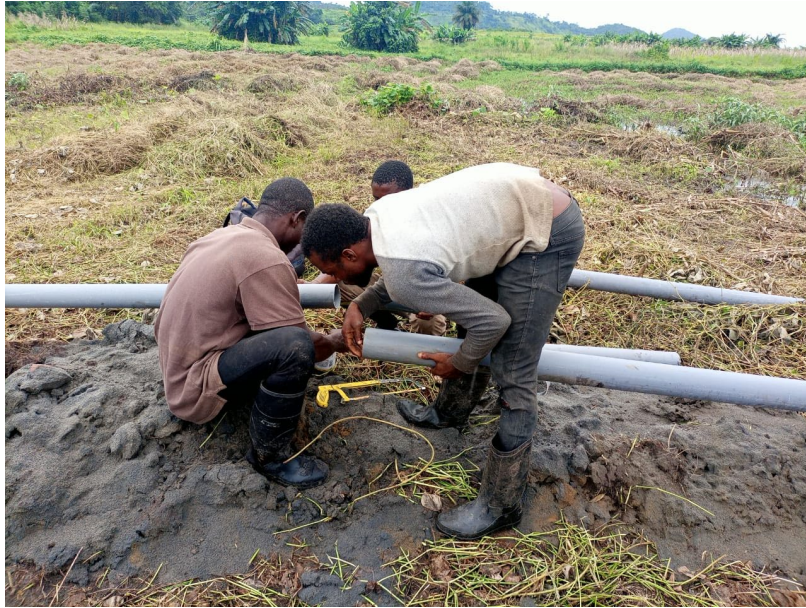
Figure 16: Jointing pipes with glue
