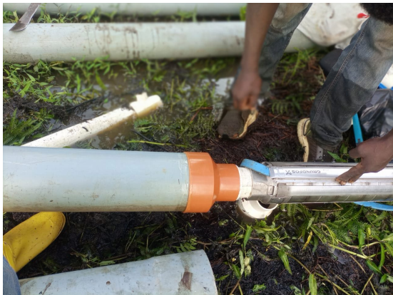
Figure 21: Connecting Solar Pump to Supply Pipeline
