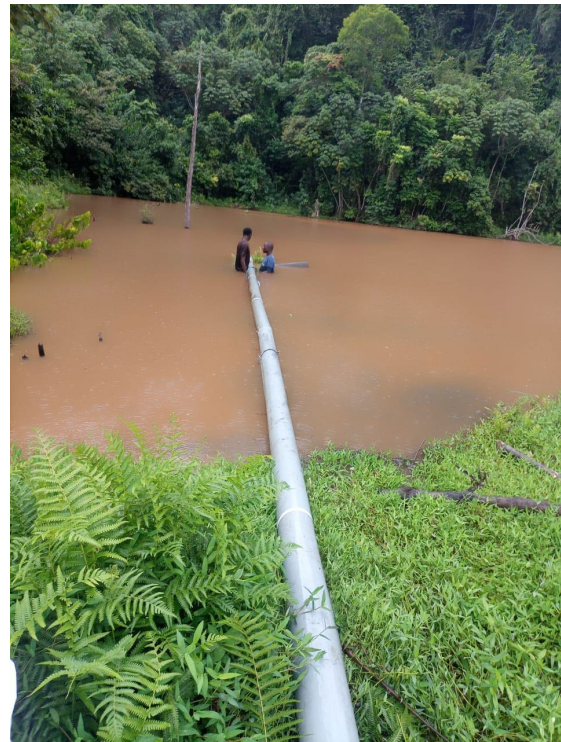
Figure 22: Lowering the Solar Pump/SP into the pond
