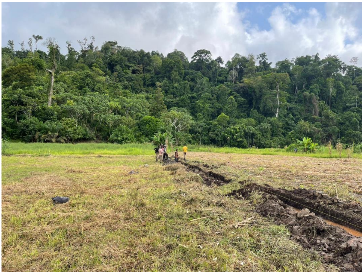
Figure 13: Part of cleared Pilot site
