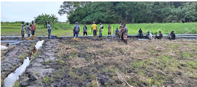
Figure 15: Laying of pipelines.
