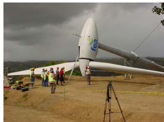
Figure 3 Fiji's wind turbine installation
