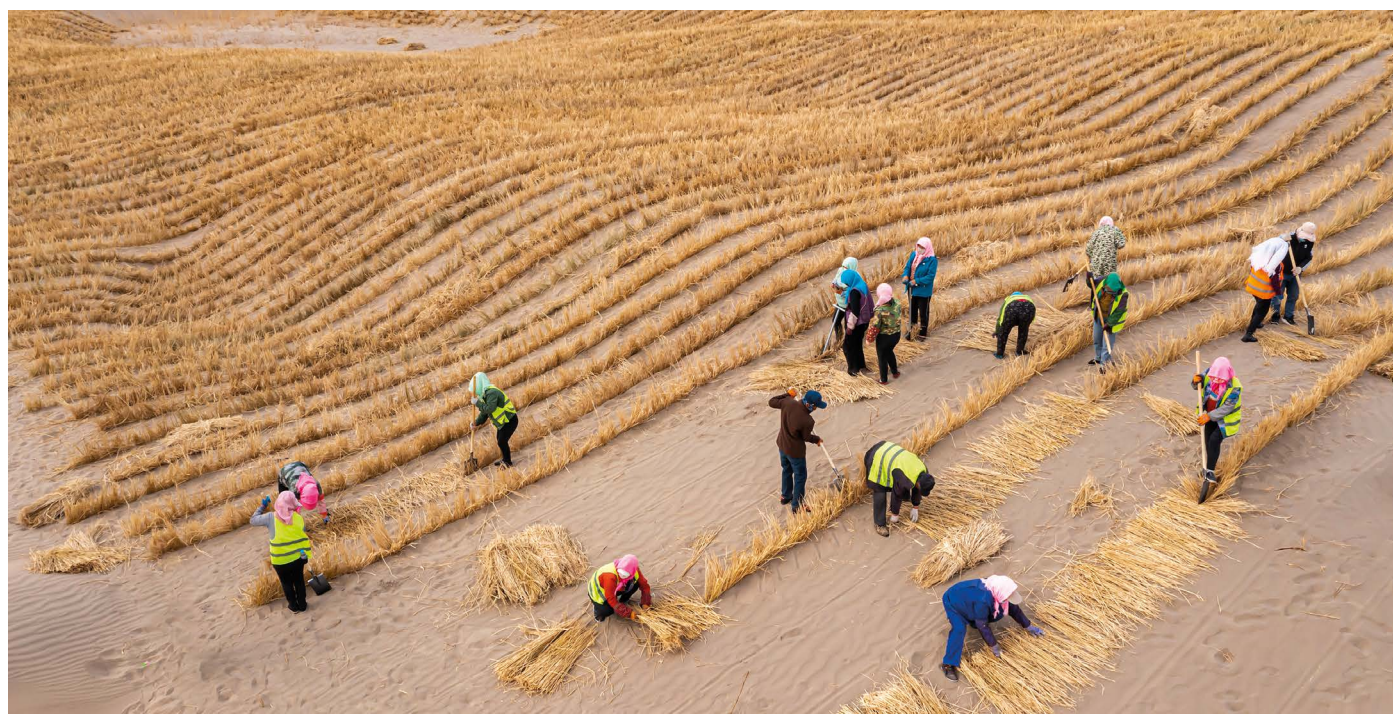
Workers plant straw barriers in desert areas in northwest China's Gansu province to stop sand from spreading, aiding afforestation.
