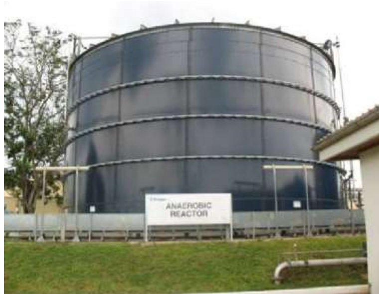
Figure 14: Biogas digester in Guinness Ghana Limited
