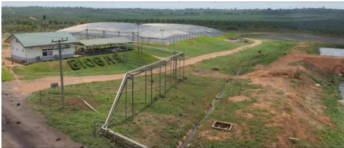
Figure 16: Biogas plant at GOPDC
